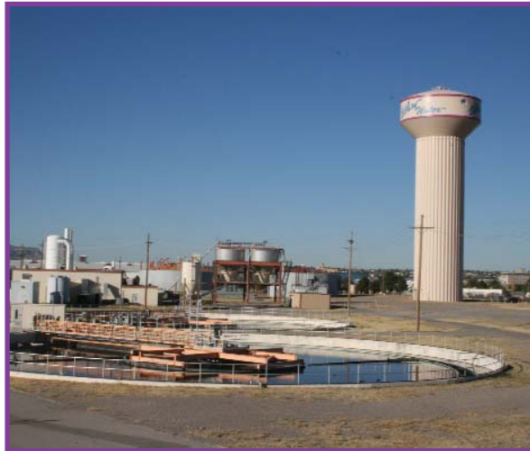
Haskell Street Wastewater Plant
